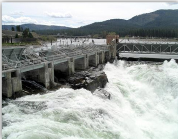
Post Falls Dam, Idaho
