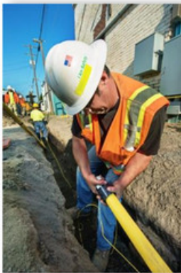
Aldyl A Natural Gas Pipe Replacement
