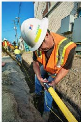
Aldyl A Natural Gas Pipe Replacement
