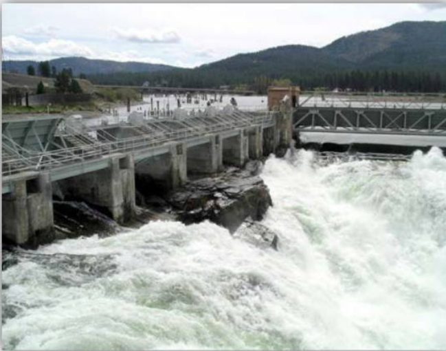
Post Falls Dam, Idaho
