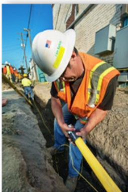
Aldyl A Natural Gas Pipe Replacement
