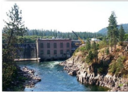
Nine Mile Falls Rehab
