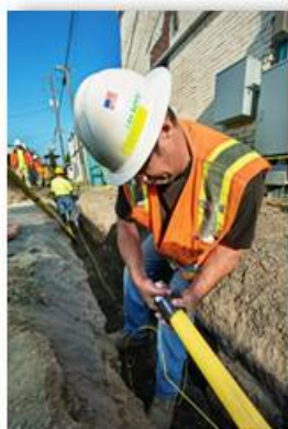
Aldyl A Natural Gas Pipe Replacement
