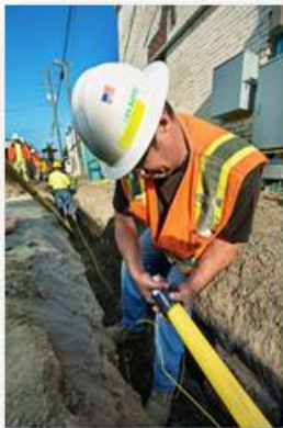
Aldyl A Natural Gas Pipe Replacement
