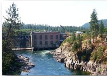
Nine Mile Falls Rehab
