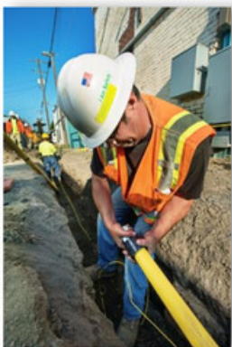
Aldyl A Natural Gas Pipe Replacement
