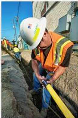
Aldyl A Natural Gas Pipe Replacement
